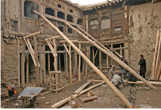
When Turquoise Mountain started working in the historic district of Murad Khani in Kabul, much of the area was buried under tons of garbage. It was placed on the World Monuments Fund Watch List of the world's most endangered sites. On the verge of collapse, the wall of this building had to be held in place with wooden props. Image courtesy Turquoise Mountain
